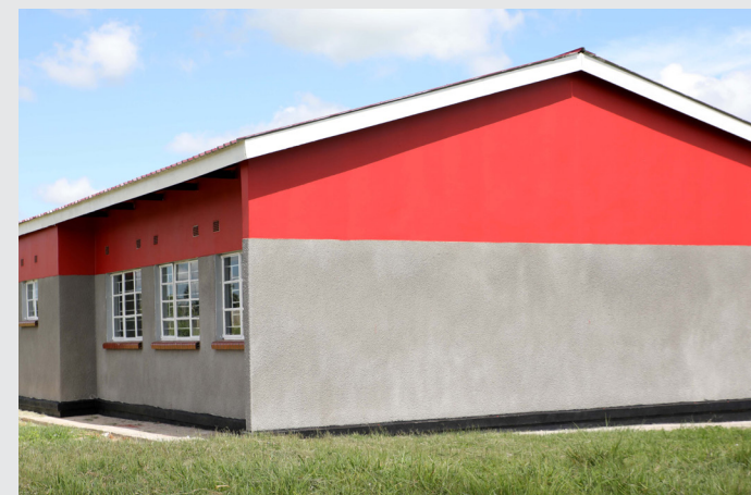
One of the donated classroom blocks at Mwalulemba Community School in Chongwe Rural worth ZMW1m.
