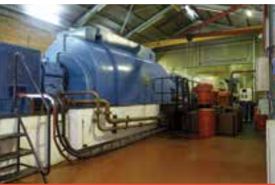
GAS TURBINE ALTERNATORS
